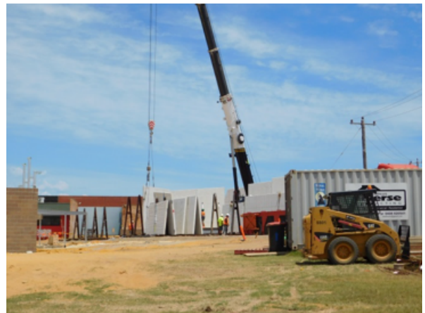
The walls to the Arts go up
